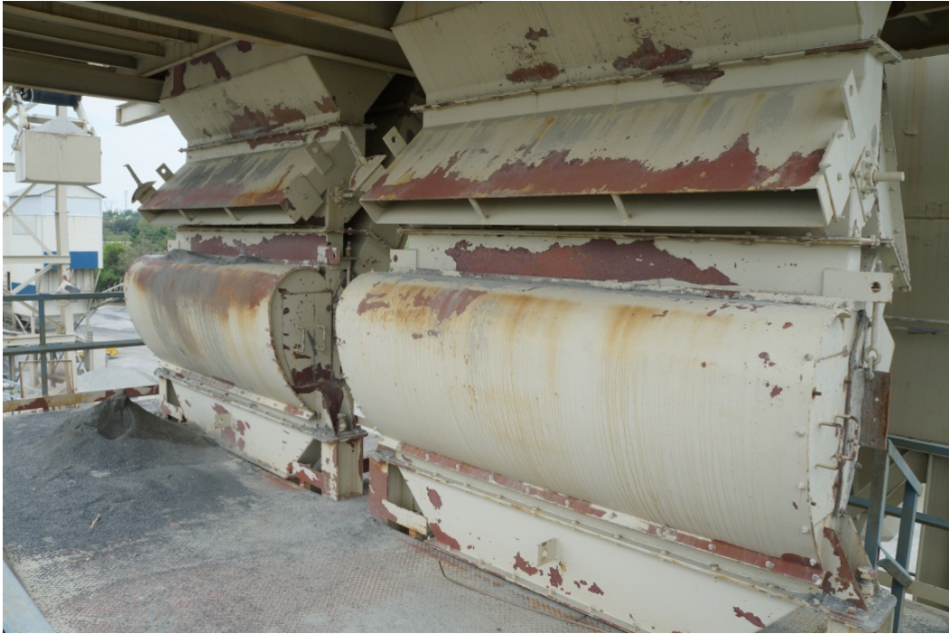
Figure 25. The dual Metso's AC22.5GI air-classifier units at Luck Stone's Goose Creek plant
