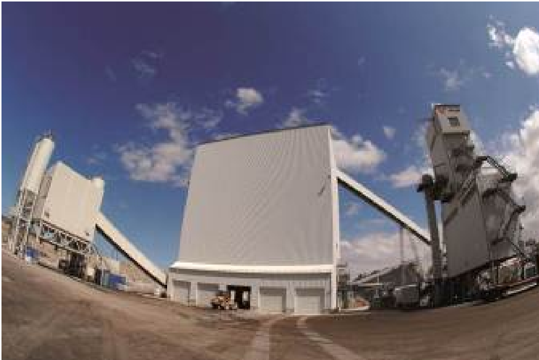
Figure 16. The centrally located silo system for storing of the 8 fractions for asphalt, concrete and industrial sand for external customers.
