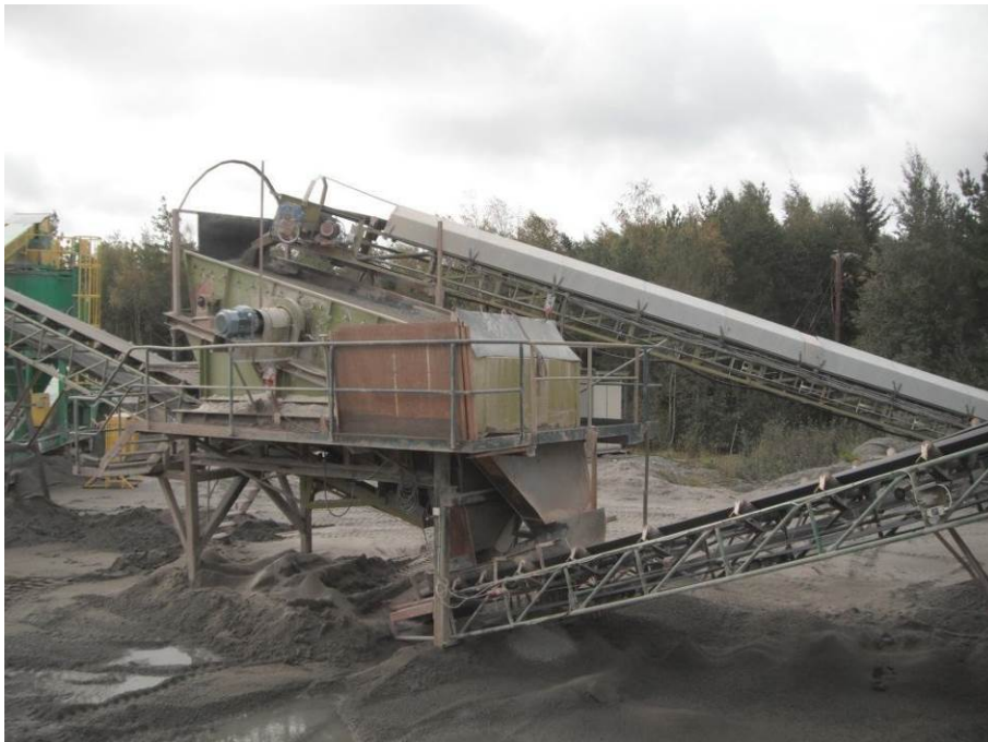
Figure 33. The screen station.
