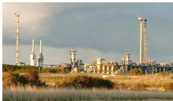
Figure 2: Existing onshore infrastructure will bring CO 2 captured in the Grangemouth cluster to the St Fergus Terminal (pictured 1 ) in the Acorn project in Scotland, UK.
