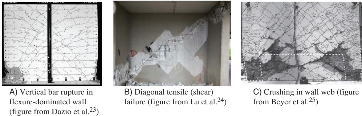
FIGURE 2 Example of damage patterns occurring in RC walls during earthquake loading
