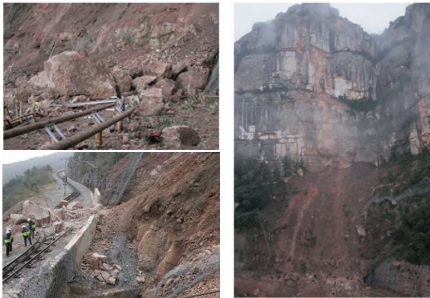
Figure 3. 2008/12/28 and 890 m 3 rockfall event at Degotalls cliff (right). In the left-hand pictures, the road and the railway cut by blocks can be appreciated.
