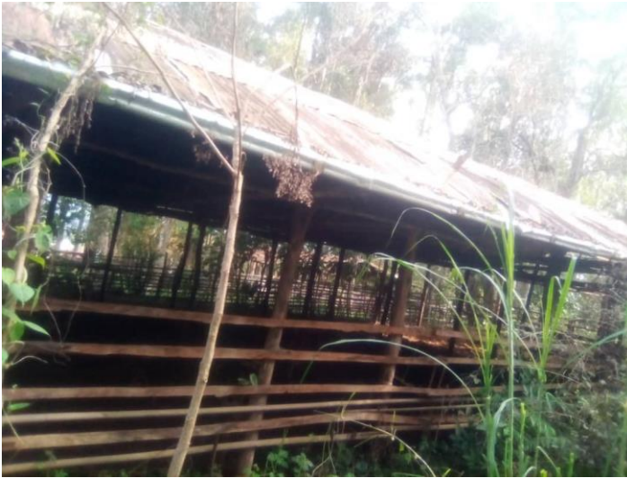
Figure 3a Type of kraals with galvanized roofing
