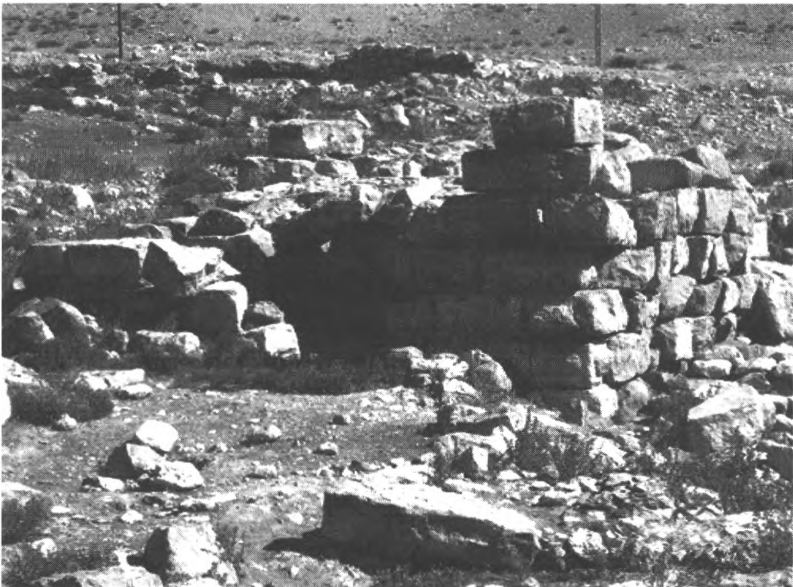
Figure 32. An arch in a building in the JIV.
