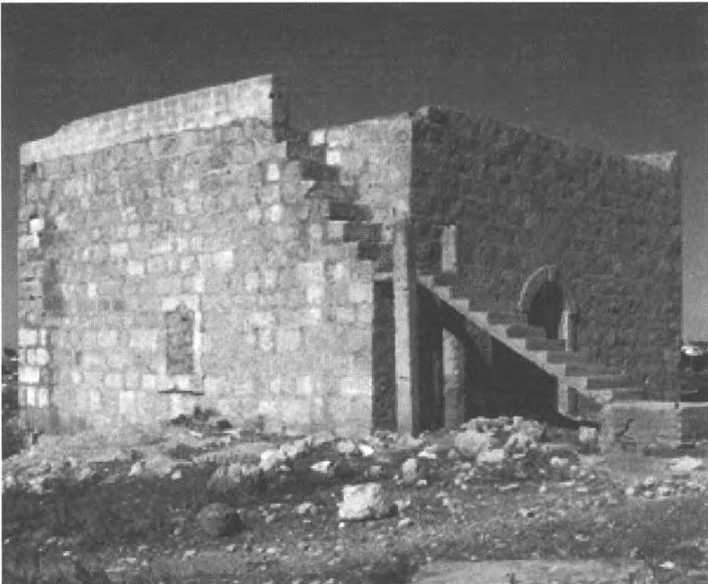
Figure 34. Building 3 in the JIV.
