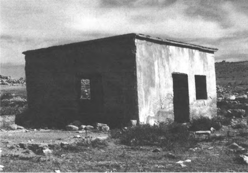
Figure 33. Building 1 in the JIV.
