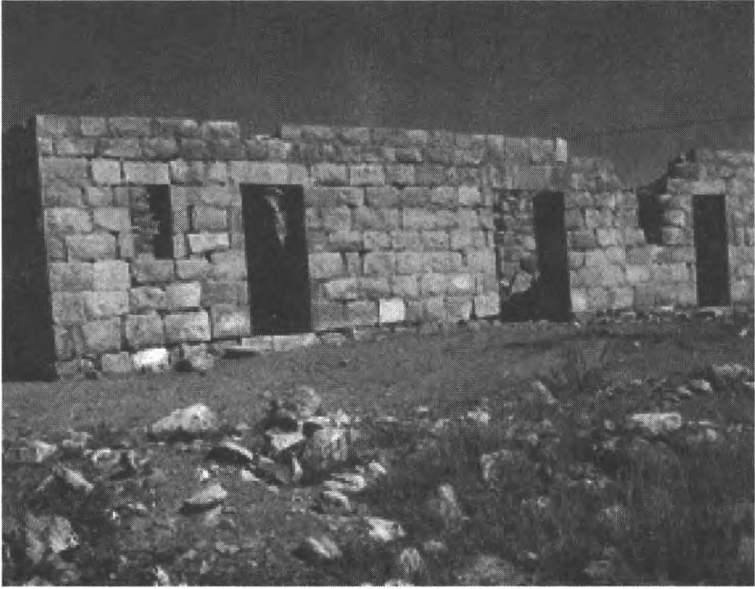
Figure 35. Building 5 in the JIV.
