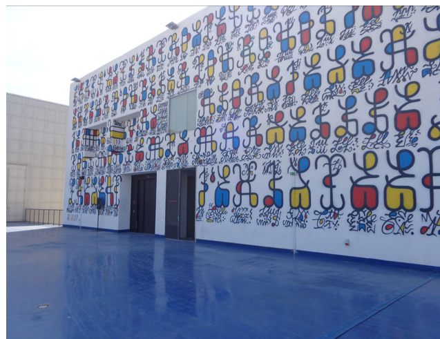
Figure 2 'Panorama'-Tower, Friche de la Belle-de-Mai Art Factory, Perimeter Euroméditerranée Credit: Mathilde Vignau
