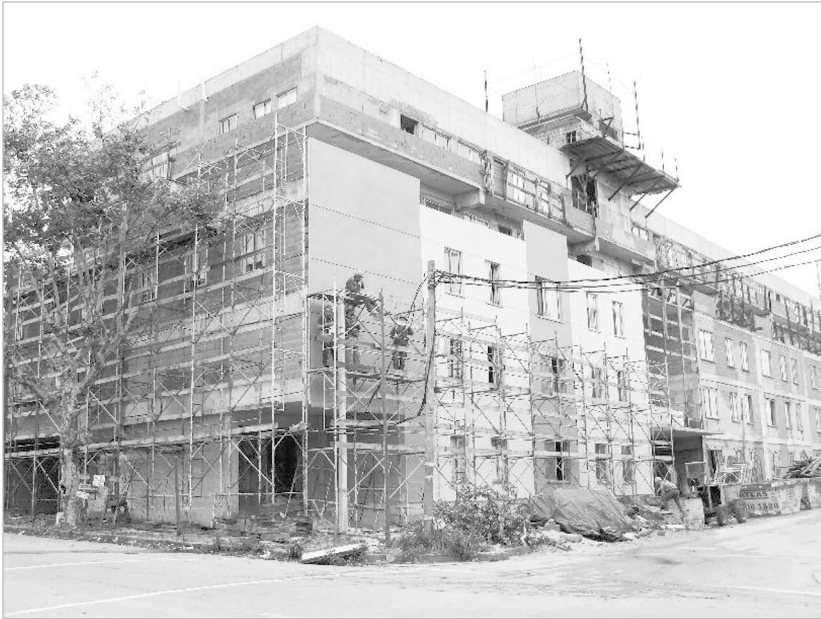
Figure 3: Housing units under construction by FUCVAM cooperatives, Montevideo.
