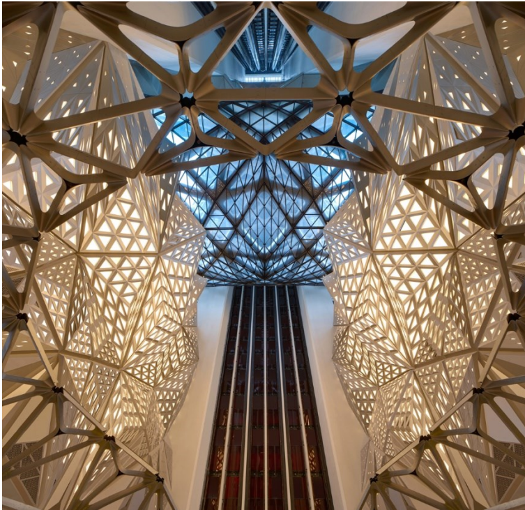
Figure 6.33. Atrium skylight of Morpheus Hotel . Photograph by Virgile Simon Bertrand. Morpheus Hotel , Zaha Hadid Architects, 2019.
