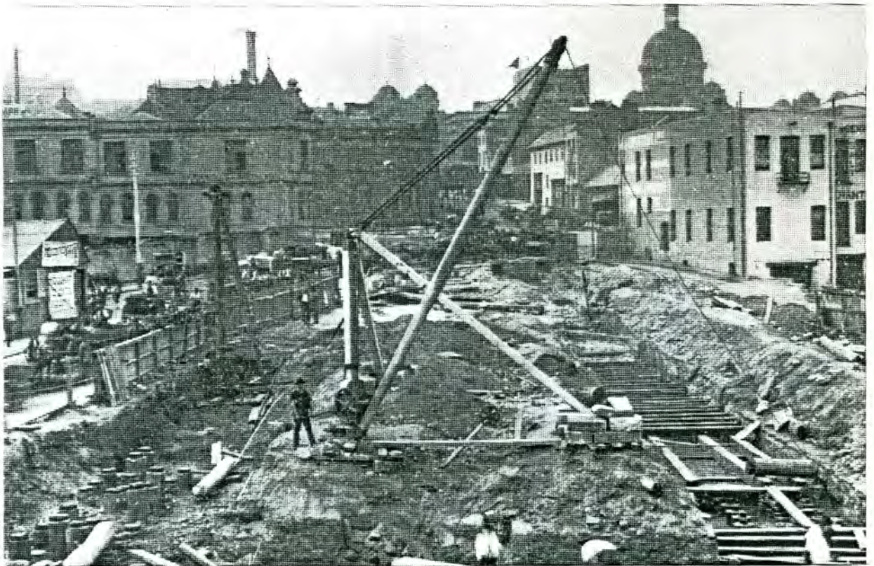
Pymont Bridge Under Construction, The Eastern Approaches, 1900. Source, DMR Archives
