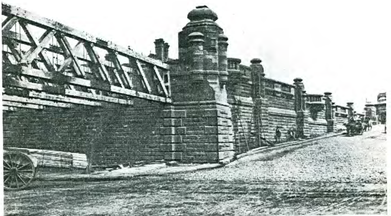
Pymont Bridge Under Construction, The Western Abutments, 1900. PLATE NO.19 Source, DMR Archives
