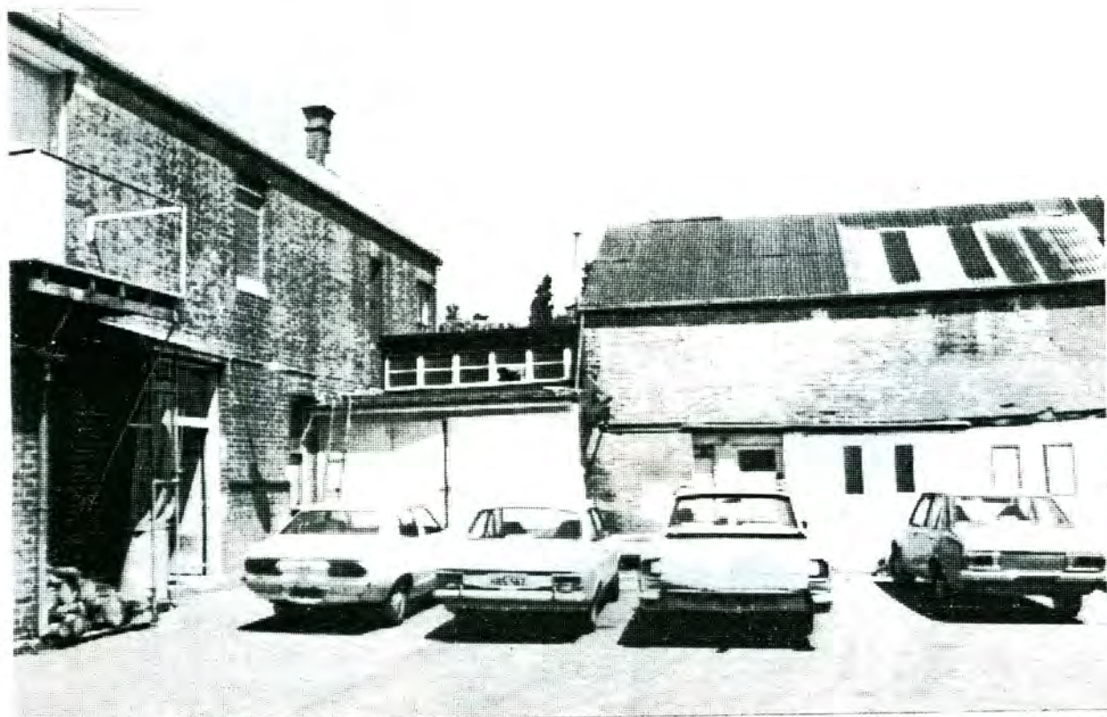
19 Duncan Street, Rear Yard, 1982.
