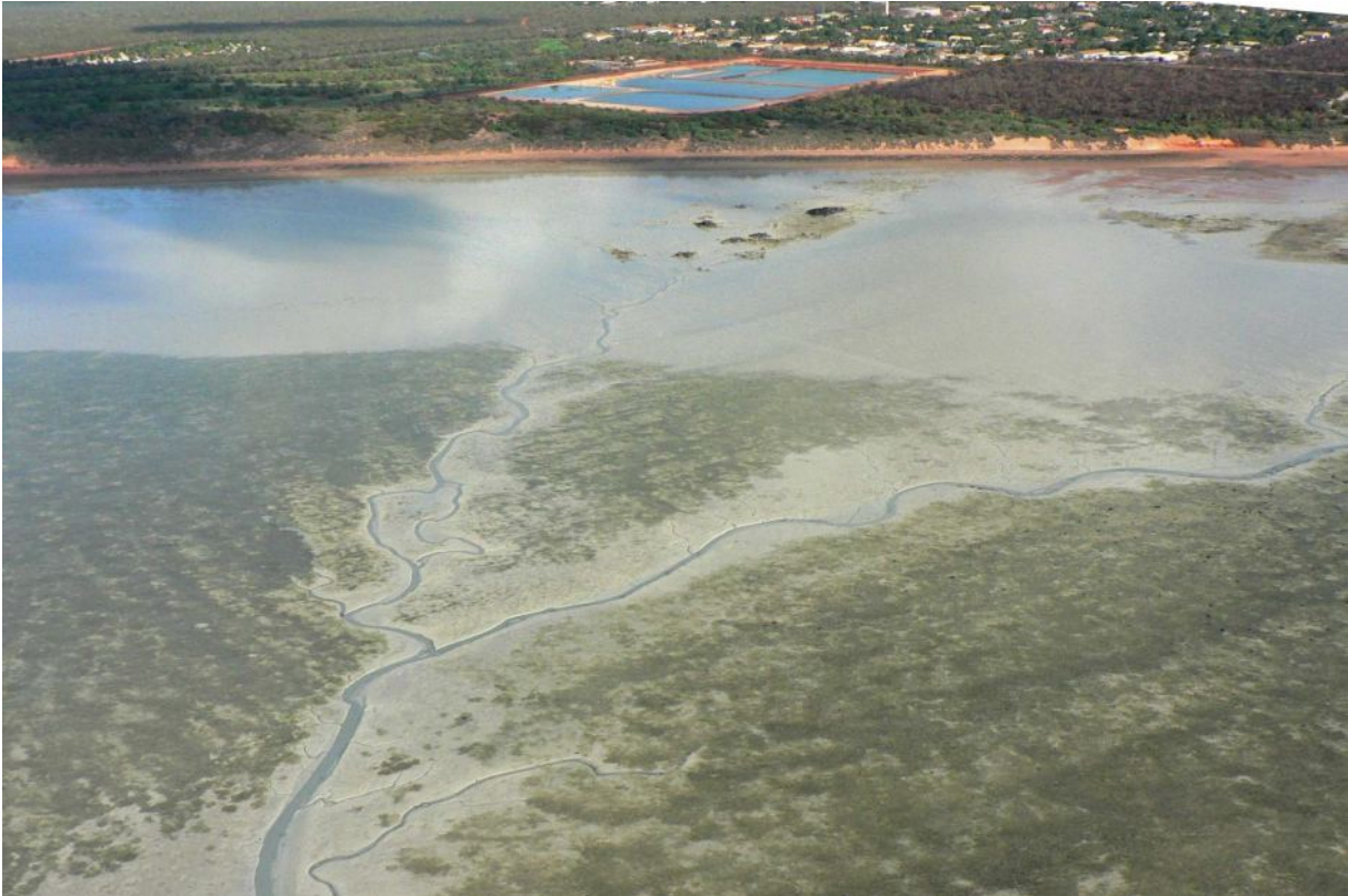
Figure 5.13. Broome Waste Water Treatment Plant (WWTP) as seen from Roebuck Bay. Broome city is to the right (east) of the picture. The golf course can be seen to the left (west) of the WWTP.
