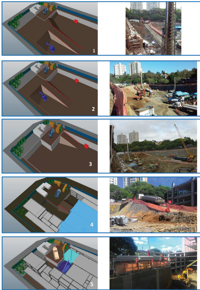
Fig. 5. Different positions of the access ramp during the project. [Colour online.]
