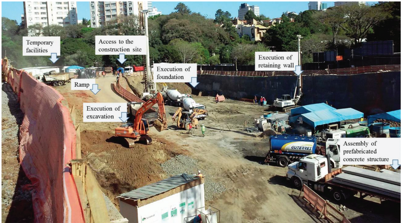
Fig. 1. Overview of the construction site. [Colour online.]
