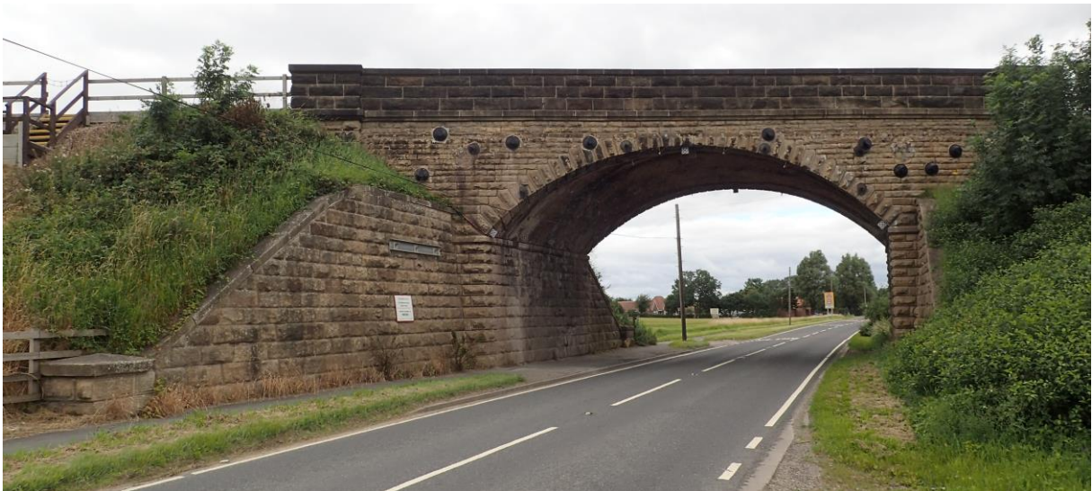
Figure 4.1: Upside elevation view of the CFM-5 bridge, looking north
