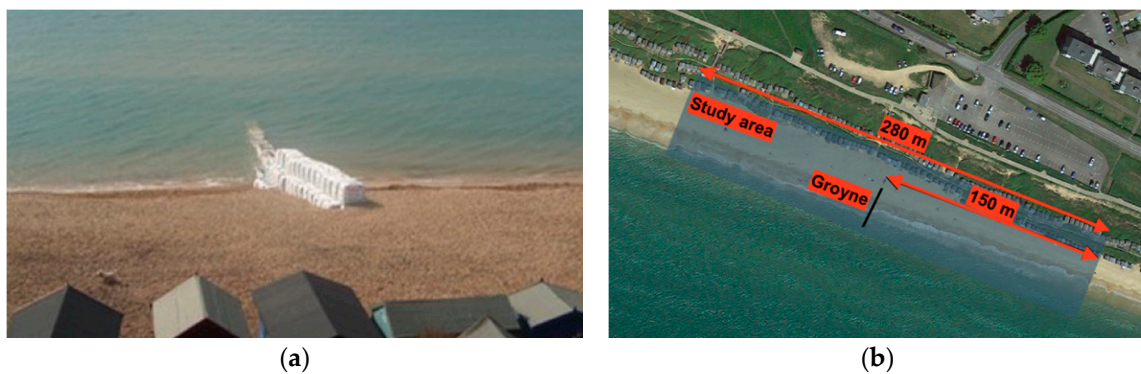
Figure 10. (a) View of the temporary structure from the top of Hordle Cliff the 6 October 2007; (b) plan view of the study site and groyne position.
