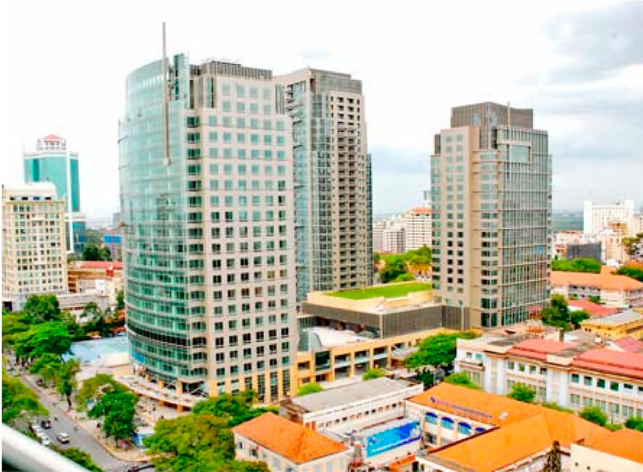
Figure 10. The Kumho Asiana Plaza: offices, apartments, the InterContinental Asiana Saigon hotel and residences. Source: https://c1.staticflickr.com/5/4056/4652668334_1ba967fea5.jpg .
