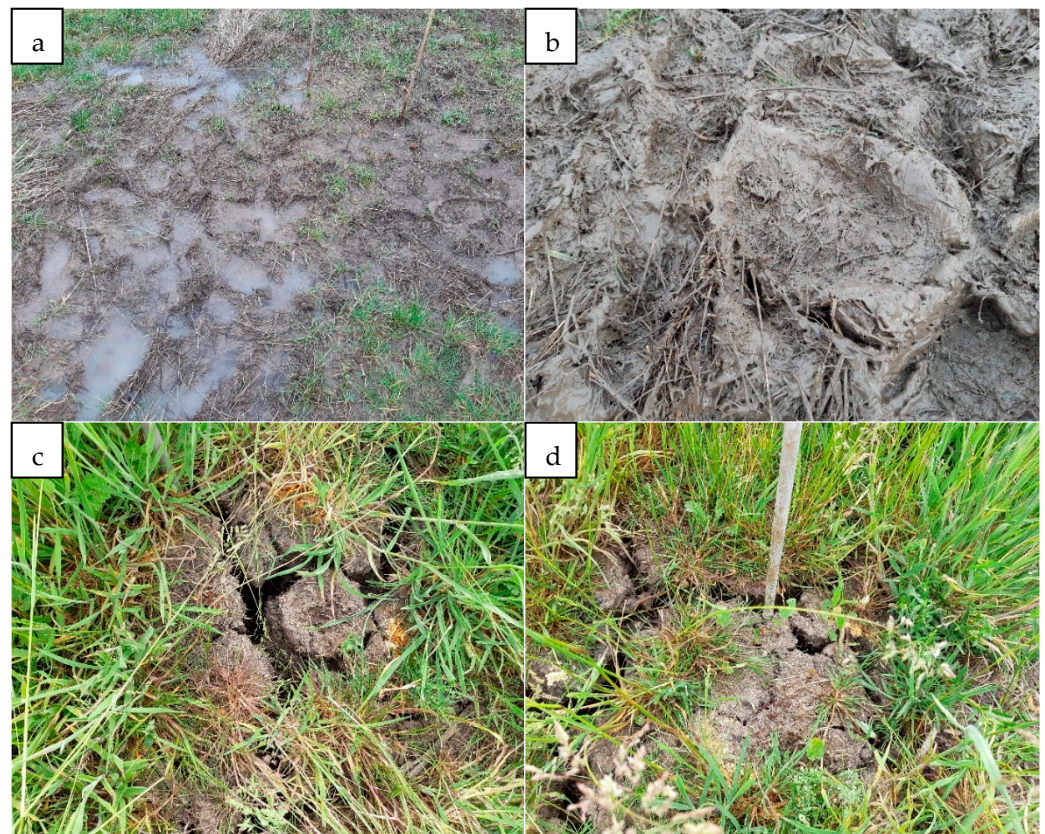
Figure 11. (a,b) saturation of the 2006 sample site during winter data collection, (c) cracking of the 2006, and (d) 2008 sample sites in the winter (locations can be identified using Figure 1).
