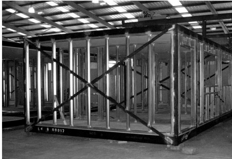
Figure 4: Corner post-module [21]
