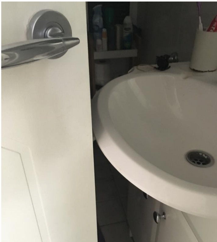
Figure 5.1: Poorly designed bathroom resulting in the door catching on the sink (Author's own photograph)
