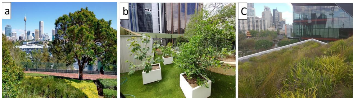
17 18 Figure 4: Examples of green roof types surveyed across Sydney—(a) Intensive green roofs, (b) roof 19 gardens and (c) semi-intensive green roofs.
