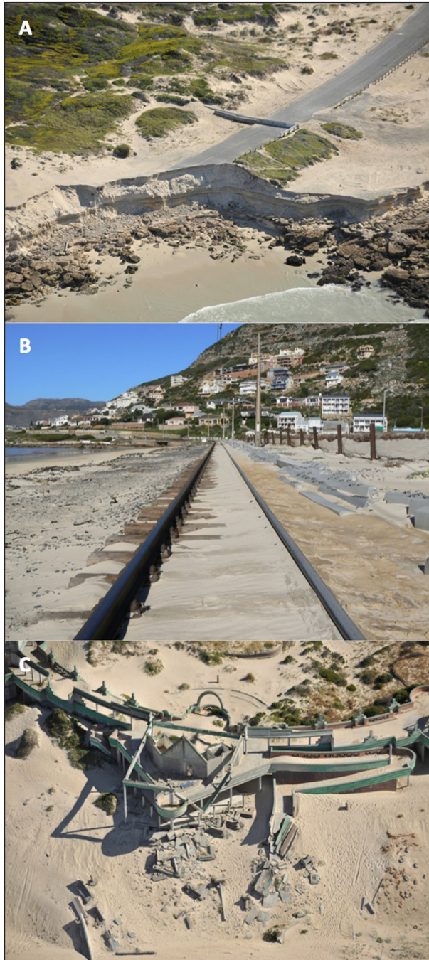
Figure 17: Examples of the coastal vulnerability of False Bay. Exposure of (A) infrastructure to erosion at Monwabisi, (B) the railway to erosion and wind-blown sand at Glencairn, and (C) broken infrastructure at the Macassar Beach coastal public resort creating an unsightly and unsafe environment (photo credits: B. Sutherland and D. Colenbrander). DOI: https://doi.org/10.1525/elementa.367.f17
