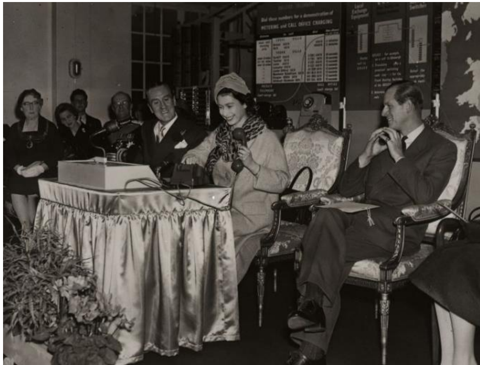
Figure 29 The Queen Opening the STD System at Bristol Telephone Exchange, 1958. 148
