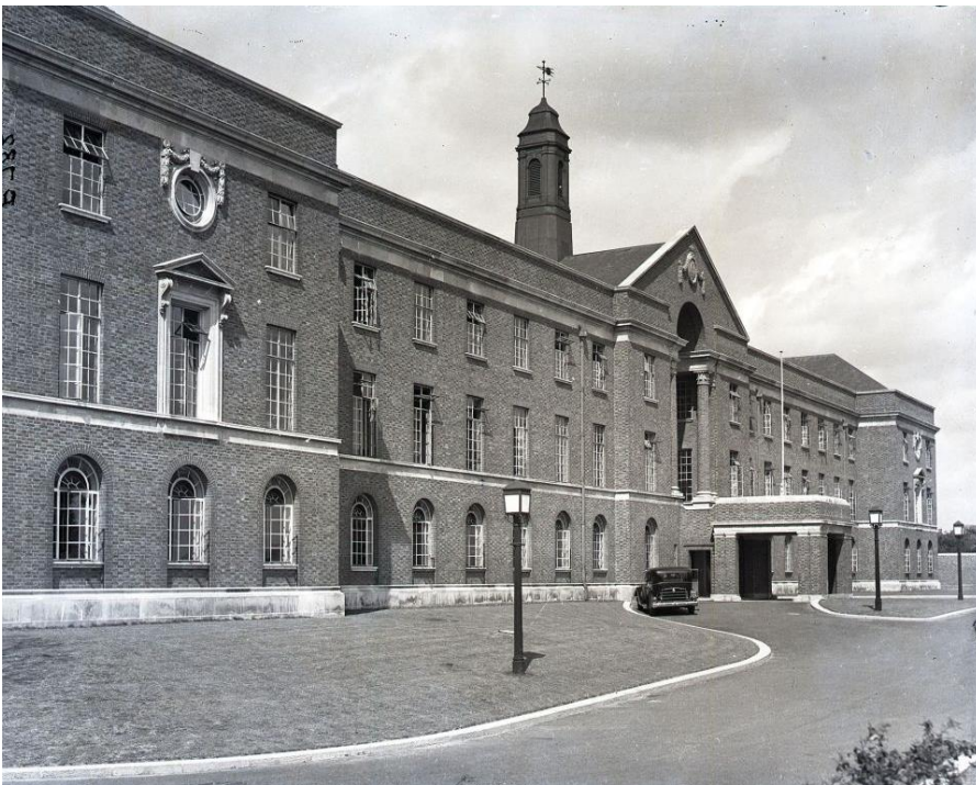
Figure 2 Photograph of the Main Research Building, Post Office Research Station, 1935. 2
