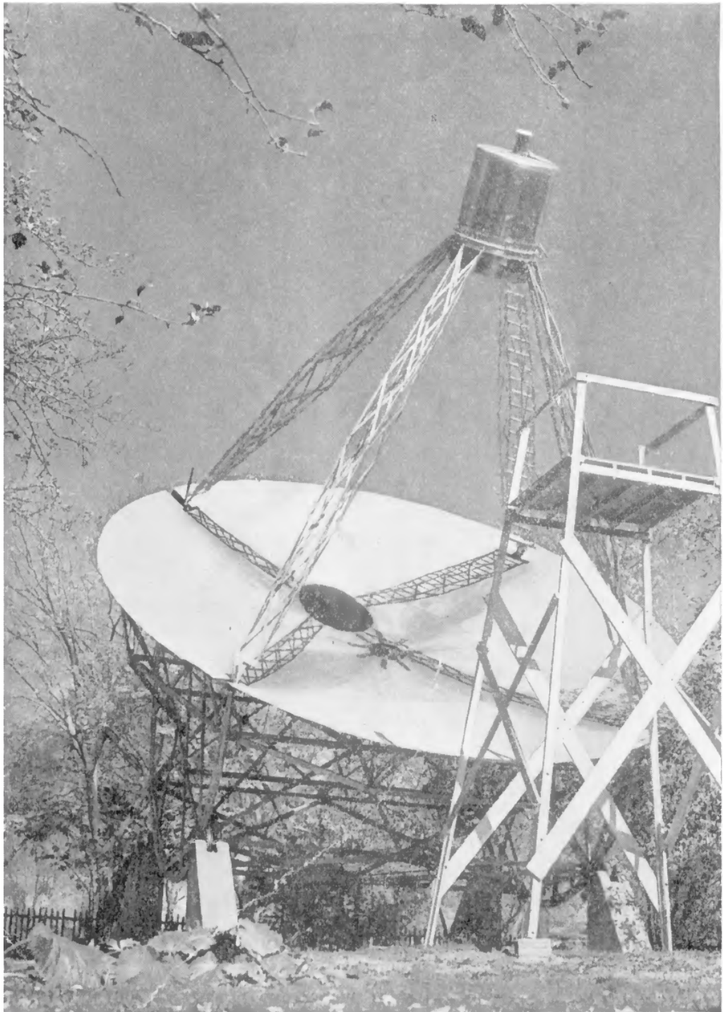
FIGURE 1.2: Photograph of the Grote Reber Telescope, Figure.1 of Reber (1944) . The Grote Reber Telescope is a sheet-metal mirror with a diameter of 31.4 feet and a focal length of 20 feet.
