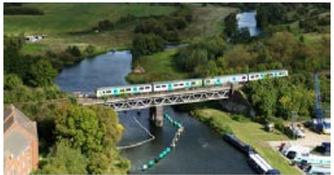
Figure 5: HydroFLEX crossing the viaduct into Evesham on a mainline test run (UoB/Porterbrook).
