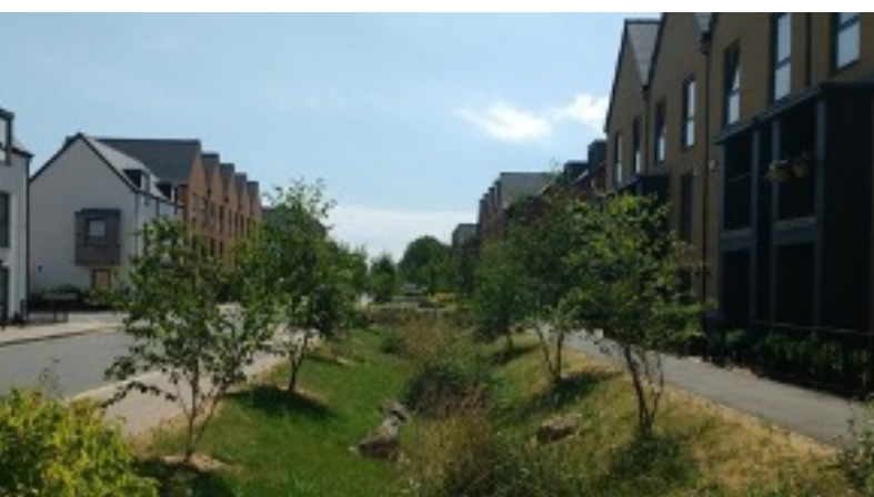
Figure 2. Award-winning SuDS designed in the recently built residential area of St. Andrew's Park in Uxbridge, the London Borough of Hillingdon. Source: Greater London Authority , Susdrain . The climate change impact of the changes required for the water sector
