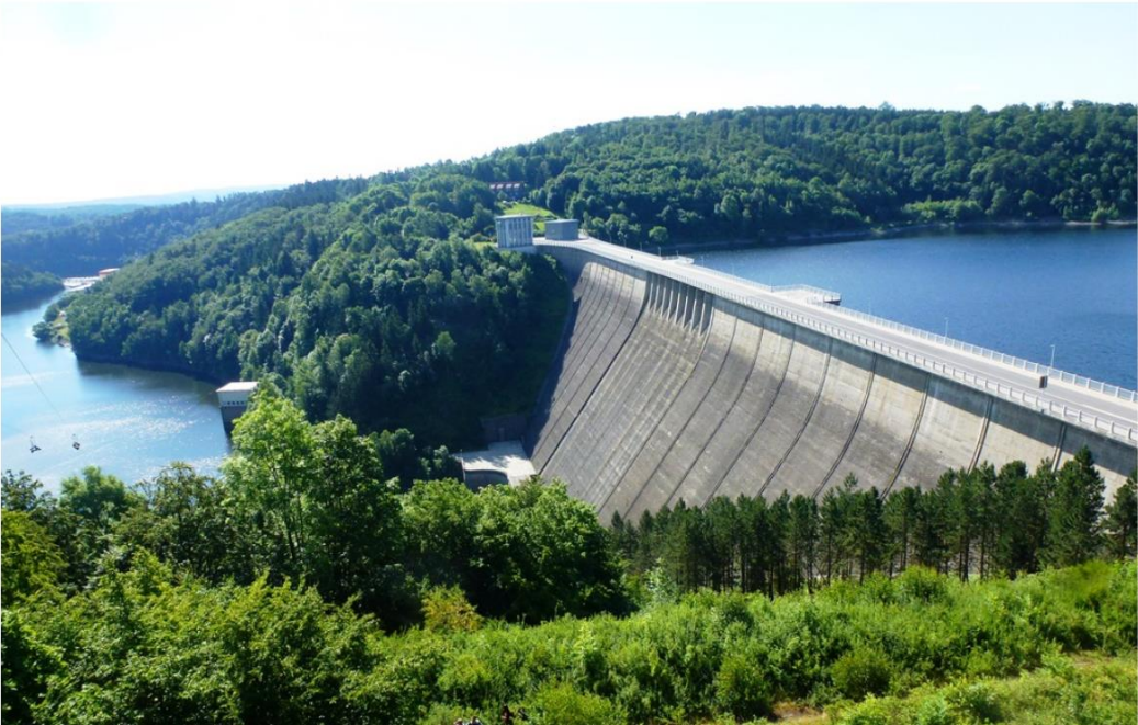
Figure 3.2: An overview of Rappbode Dam (Photo by Regional Association Harzer Urania e.V.)
