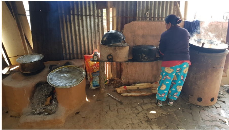
Fig. 5. TLUD condition in 2019 after 1 year of use - school kitchen P1 (colour).
