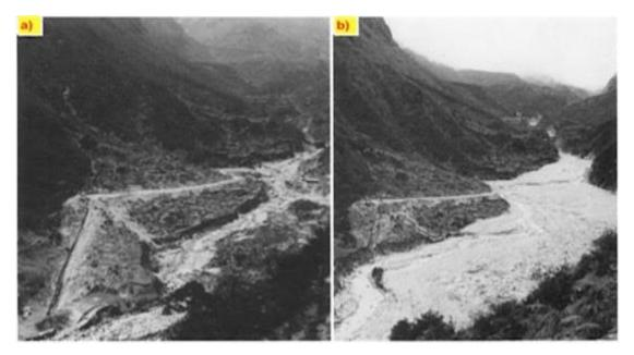
Figure 4.5 Thame Hydropower Project a) before the GLOF on 4<sup>th</sup> April 1985 and b) after the GLOF on 10<sup>th</sup> October 1985 (Vuichard, 1987)
