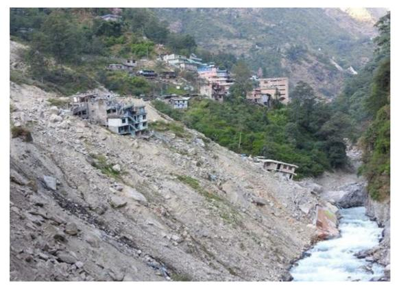
Figure 3.23 Aftermath of a landslide near Tatopani, Nepal, triggered by July 2016 GLOF at Bhote Koshi, Nepal (Kornei, 2020)
