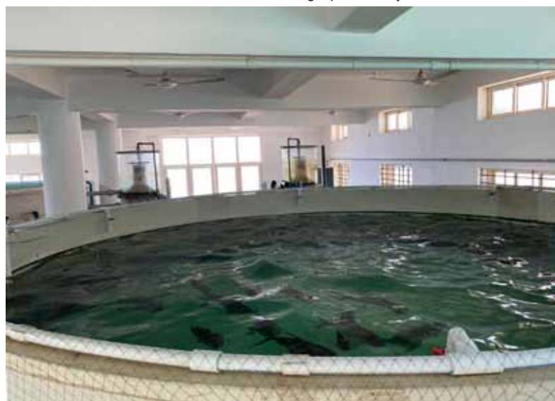
Broodstock in 30t RAS tanks
