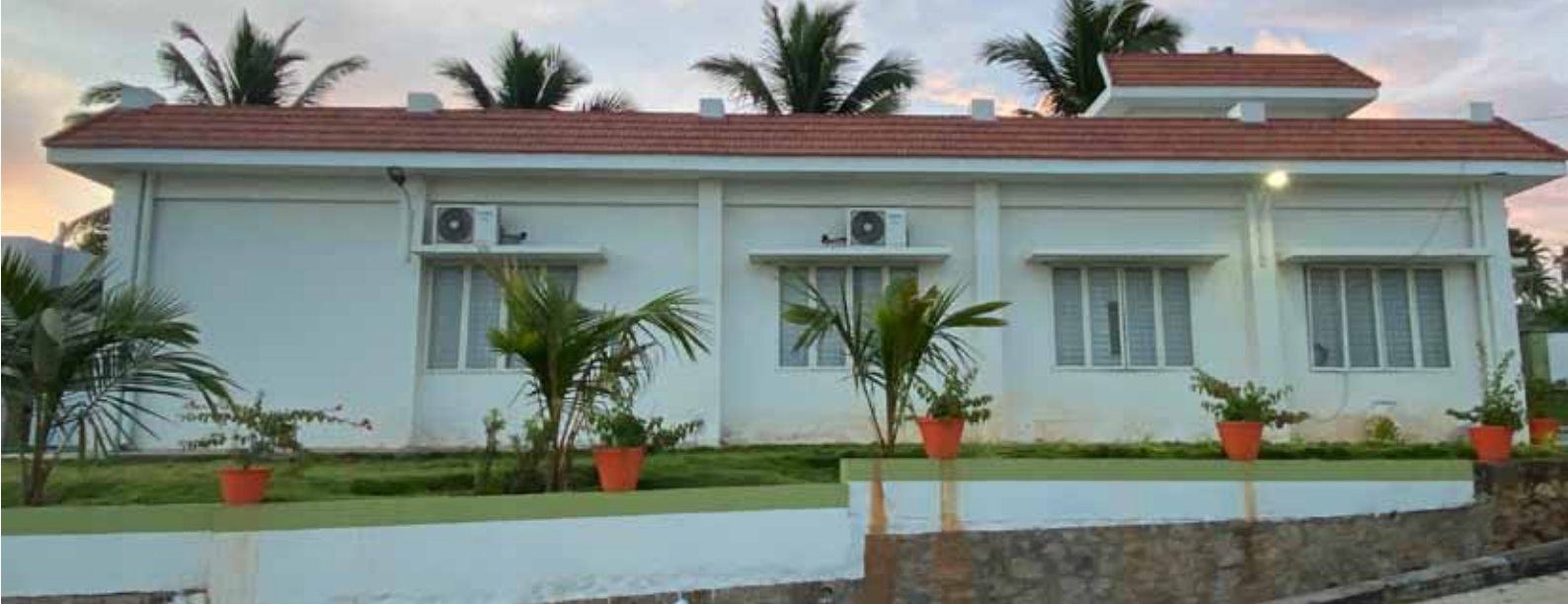
Office and Laboratory Building
