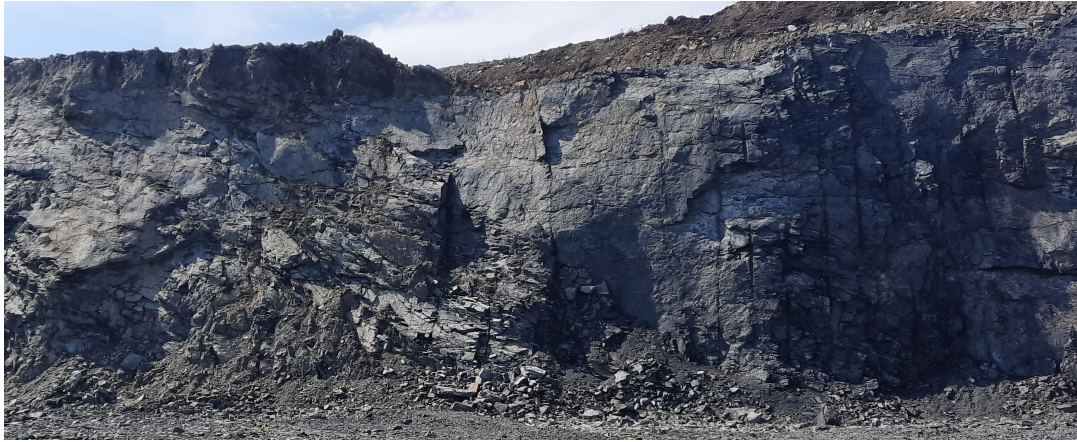
Figure 31: Photo showing an overview of the second part of the presplit wall in the first test in black schist (BS 1.2).
