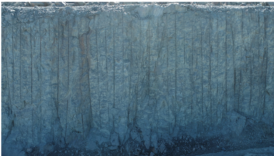
Figure 14: Presplit face from 89 mm diameter presplit holes.
