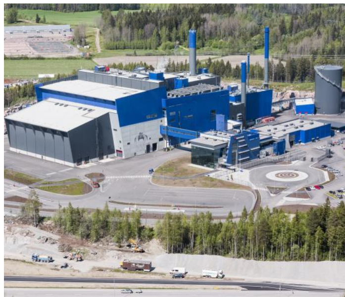
Figure 9: Vantaan Energia thermal power plant in Vantaan, Finland. Figure obtained from [87].
