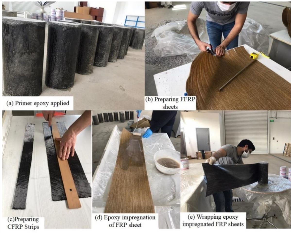
Picture 3.4 FRP confinement procedure
