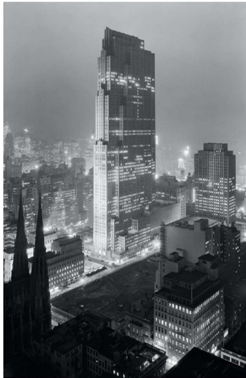
Figure 8: Construction progress of the Comcast building in December, 1933.
