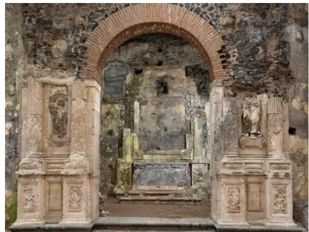
Figure 8: Entrance to the chapel of the Crocifisso in its current state. Photo by G. Sciacca.
