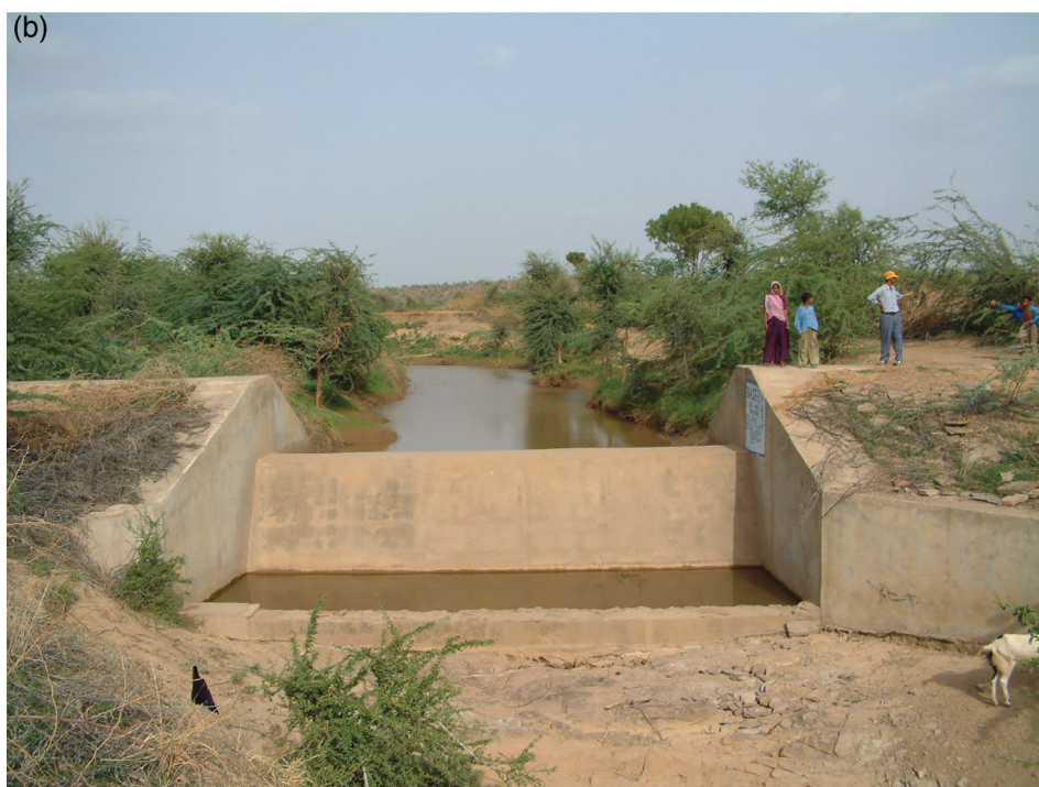
Figure 2. The village tank constructed for harvesting runoff using (a) masonry and earthen embankments and (b) check dam on a stream.
