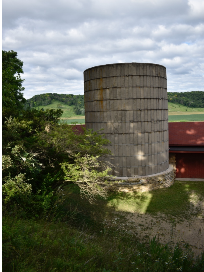
Figure 17: The original silo taken from above the hill near the Upper Cottage (left) and bird-eye view looking down at the silo (top). The interior wooden in-lining is collapsed. Image by Author, 2020 (left); courtesy of University of Pennsylvania Center for Architectural Conservation, 2020 (top).
