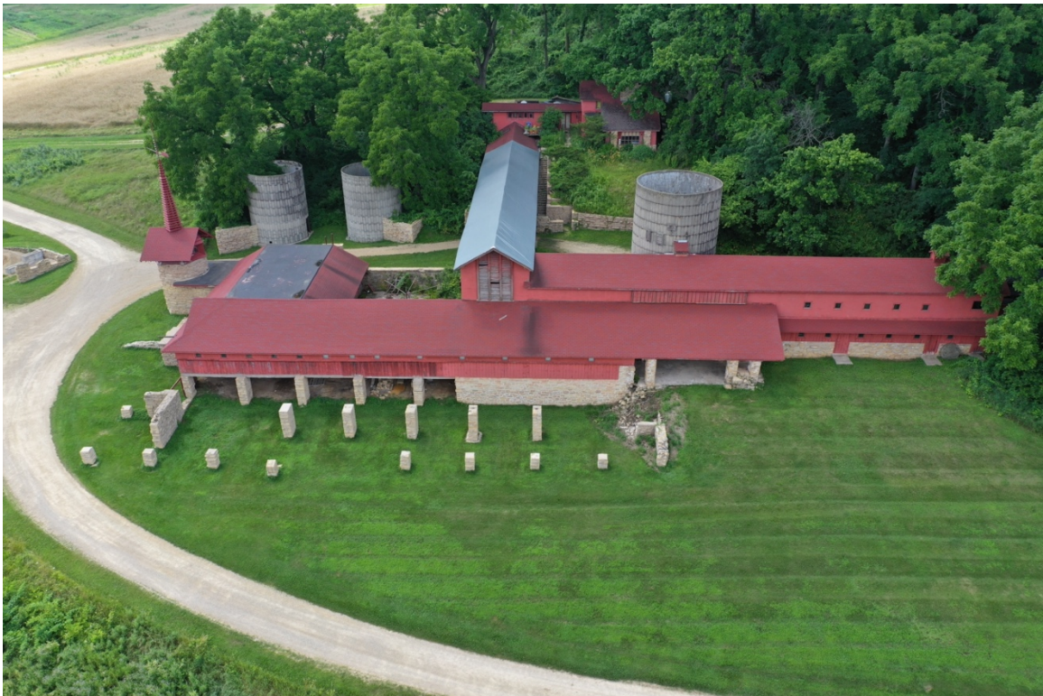
Figure 20: Drone aerial image looking westward to Midway Barn. The louvers of the hayloft and the ventilator board near the original silo provided natural ventilation. Courtesy of University of Pennsylvania Center for Architectural Conservation, 2020.
