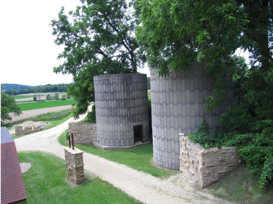
Figure 9: The “twin” concrete stave silos near the southern end of the barn. Image by Author, 2020.
