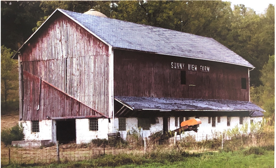
Figure 16: The north end of Midway Barn with a pentroof over the calf pen on the lower level (top) and a Swiss barn with a pentroof in Green County, Highway 62 and Old Highway 62 north of New Glarus, Wisconsin, date unknown from Barns of Wisconsin (Madison, WI: Wisconsin Historical Society Press, 2010), 36 (Bottom). Image by Author, 2020 (top) and courtesy of Steve Apps (bottom).
