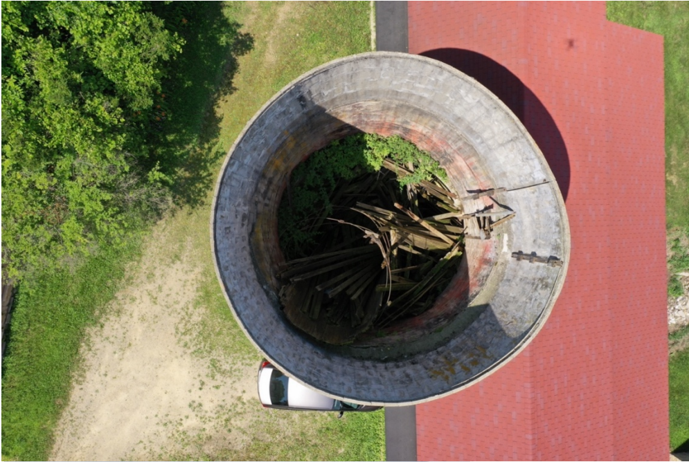
Figure 17: The original silo taken from above the hill near the Upper Cottage (left) and bird-eye view looking down at the silo (top). The interior wooden in-lining is collapsed. Image by Author, 2020 (left); courtesy of University of Pennsylvania Center for Architectural Conservation, 2020 (top).
