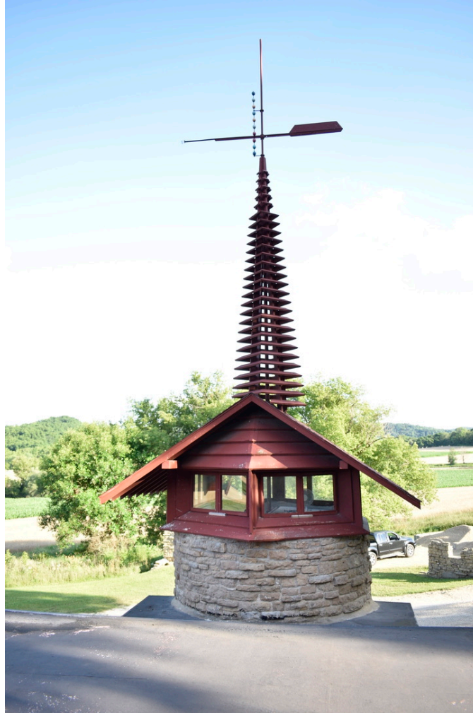
Figure 10: The upper part of the milk tower with the glass-walled bedroom and the spire with the weathervane. Image by Author, 2020.
