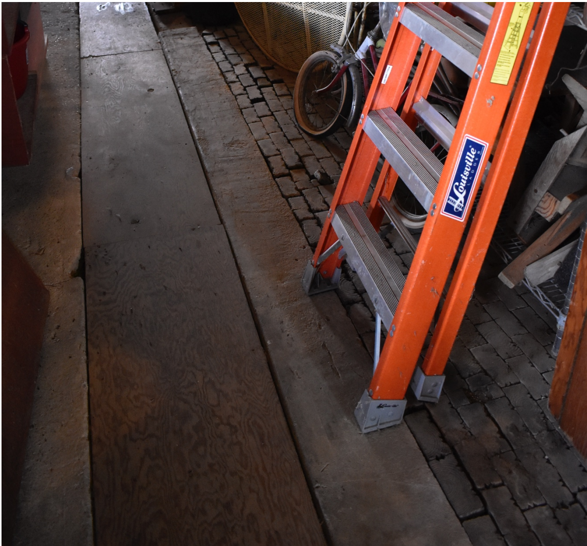
Figure 18: Wood overlay and wooden block insets in the floor of the flat-roof cow barn. Image by Author, 2020.
