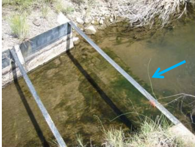
Figure 2. Moss growth on the entrance to the Parshall flume in the S.A.B. Canal
