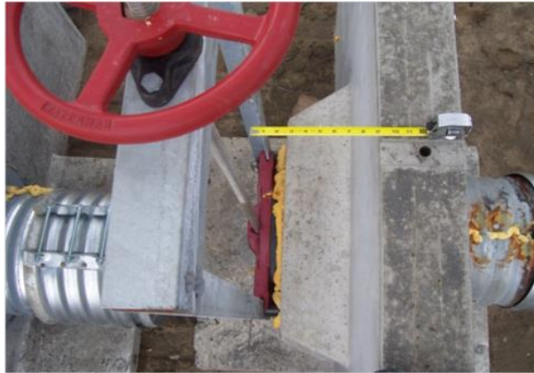
Figure 18. Example of a stilling well with too small of a diameter. The operators will not be able to see the water surface and severe surging (up and down movement) will occur.
