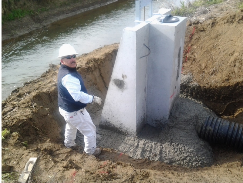
Figure 21. Field installation of a pre-cast canal metergate (Glenn Colusa ID)
