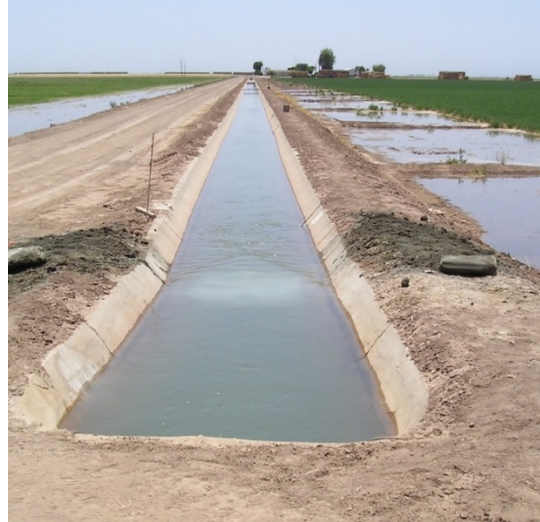
Figure 1. Field ditch with “bump” visible below the water surface near the head of the canal. This is the first irrigation set, with the area closest to the supply canal being irrigated first. The “bump” barely creates a ripple on the water surface.
