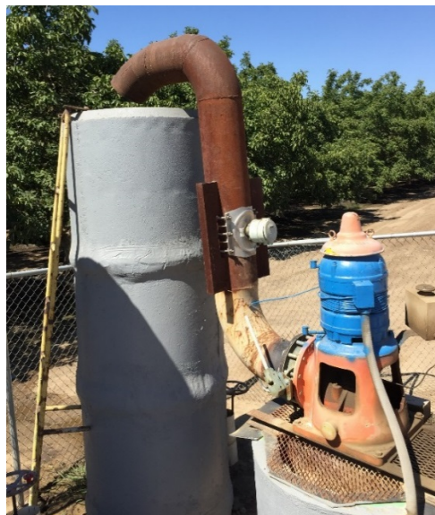
Figure 4. Propeller meter with a vertical orientation
