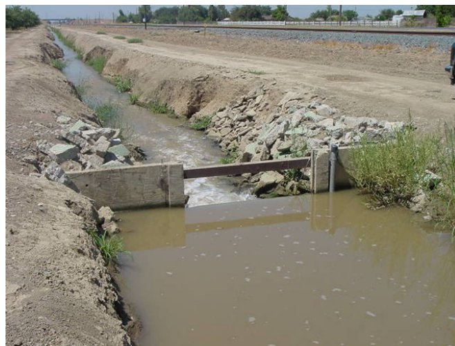
Figure 44. Example of a rectangular contracted weir
