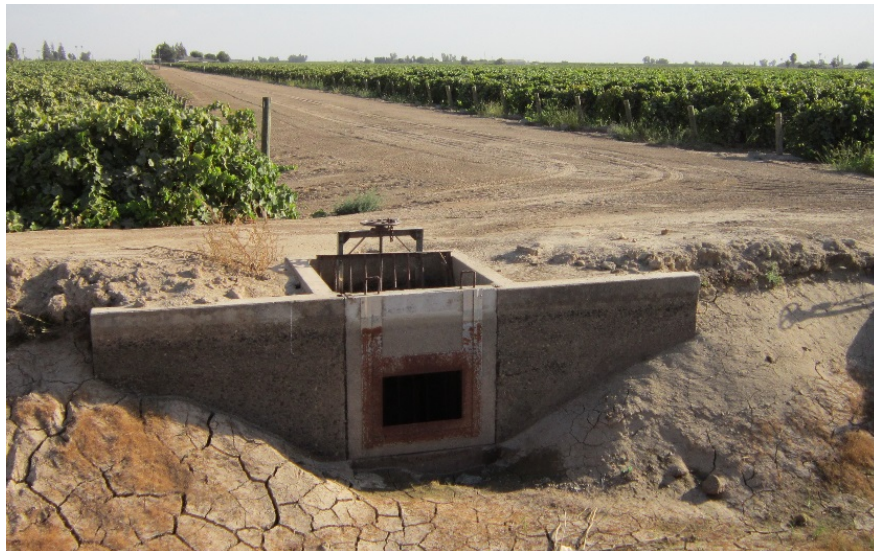
Figure 25. A fixed contracted submerged rectangular orifice at Fresno ID
