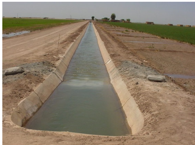
Figure 2. Same ditch. The irrigated area, and check dam, have been moved downstream in the farm ditch. The “bump” has kept the water level in the first part of the ditch high – helping to ensure that the flow rate into the ditch remains fairly constant.
