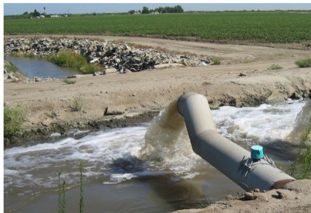
Figure 6. An elbow installed downstream of a propeller meter. In this case, the elbow is much higher than it needs to be. It only needs to be high enough to make the pipe completely full.
