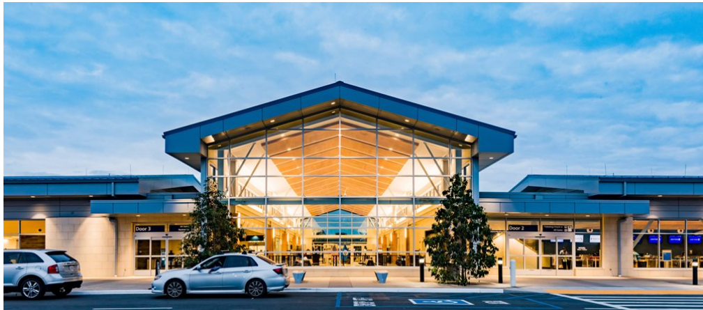
Figure 3: San Luis Obispo Regional Airport terminal (San Luis Obispo Regional Airport, 2020)
