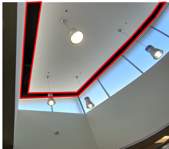
Figure 52. Smoke extraction system, highlighted in red.
