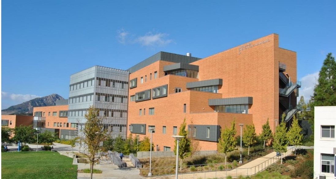
Figure 2. South side of Baker Science.
