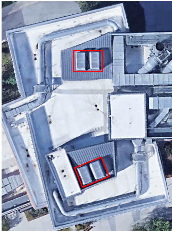
Figure 45. Smoke control vents highlighted in satellite view.
