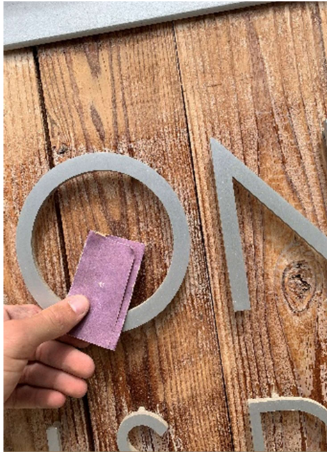
Figure 5- Hand Sanding Between and Behind Metal Letters
