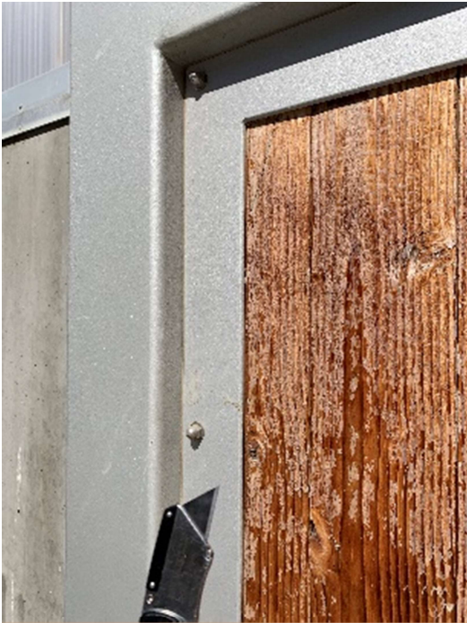
Figure 1 – Utility Knife Cutting exterior Sealant
