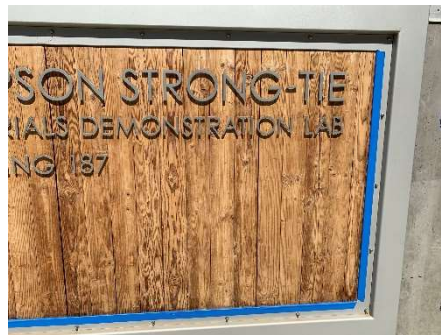
Figure 8- Taping Prior Application of Stain
