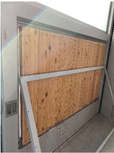
Figure 2- Removal of Interior Metal Frame/ Identification of Horizontal Bolts
