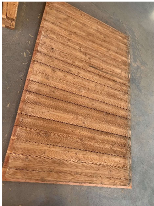
Figure 4- Existing Stain Removed From Left-Hand Panel
