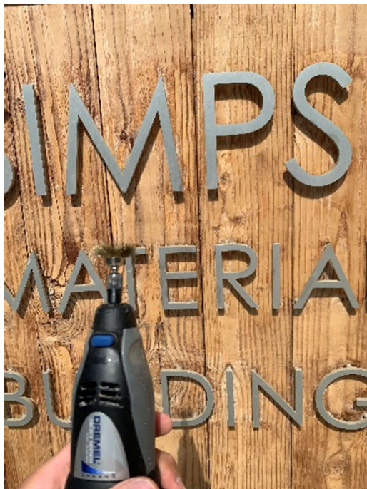
Figure 6- Use of Dremel to Remove Stain Behind/ Between Letters
