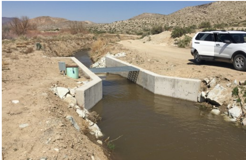
Figure 8. Concrete Replogle flume built in a rectangular cross-section on High Canal
