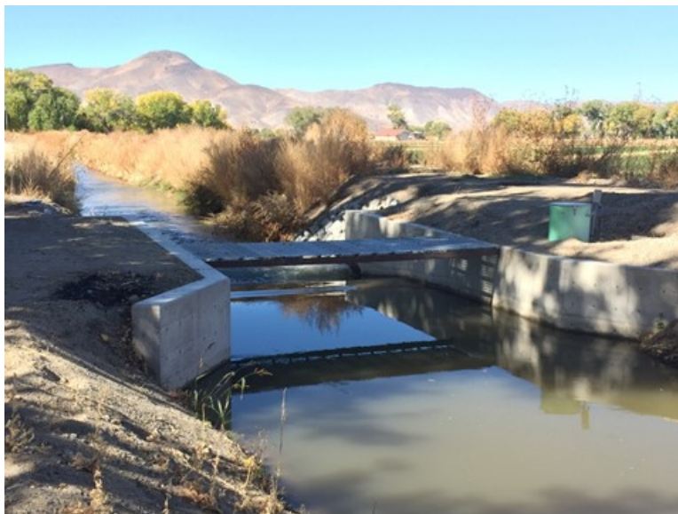
Figure 14. Replogle flume on Fox Mickey Canal
