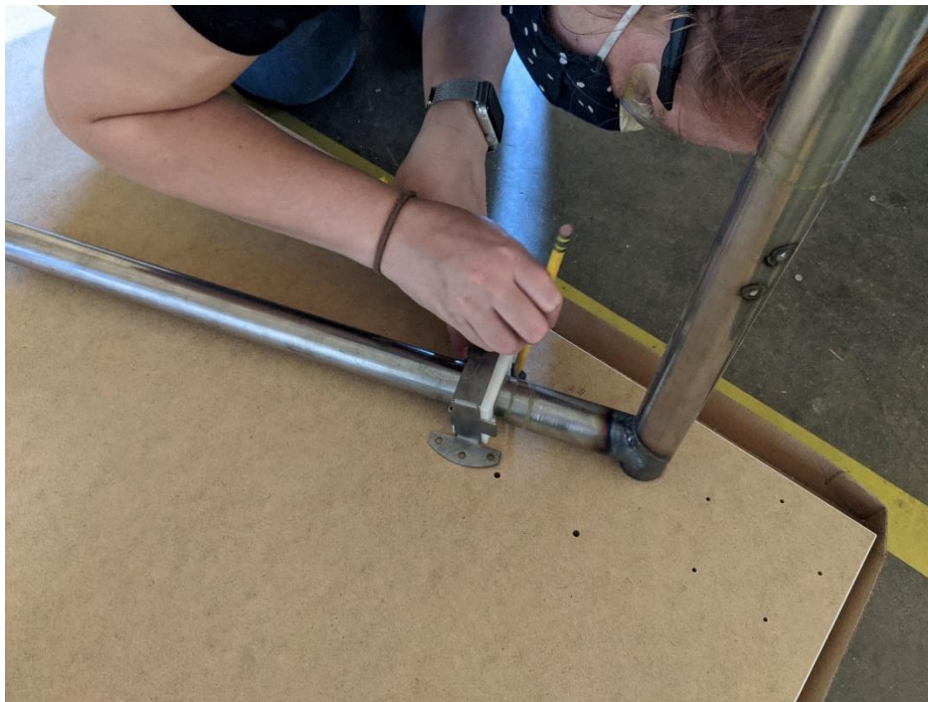
Figure 59: Locating the holes for wood anchors.
