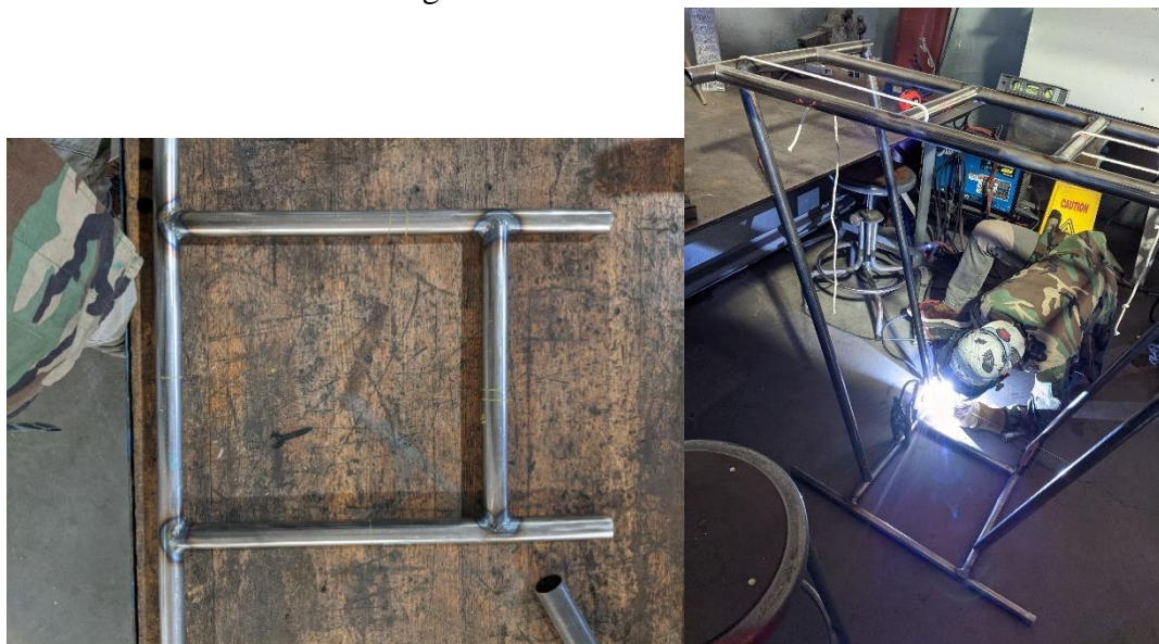
Figure 57: Snapshots of frame welding process.
