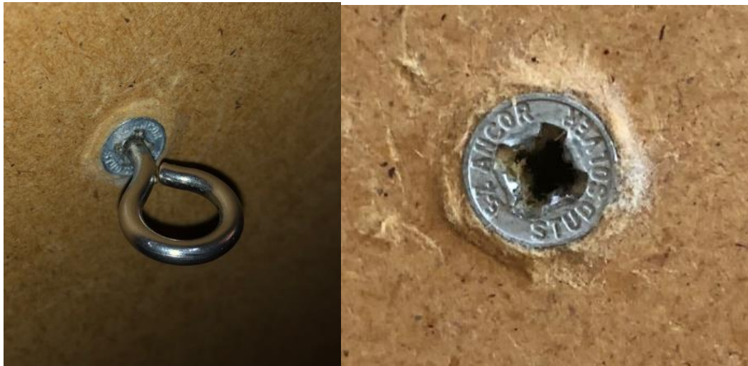
Figure I11: EZ Ancor installed with adhesive.
