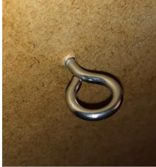
Figure I8: Bare Screw eye hardware installed in a pre-drilled hole.
