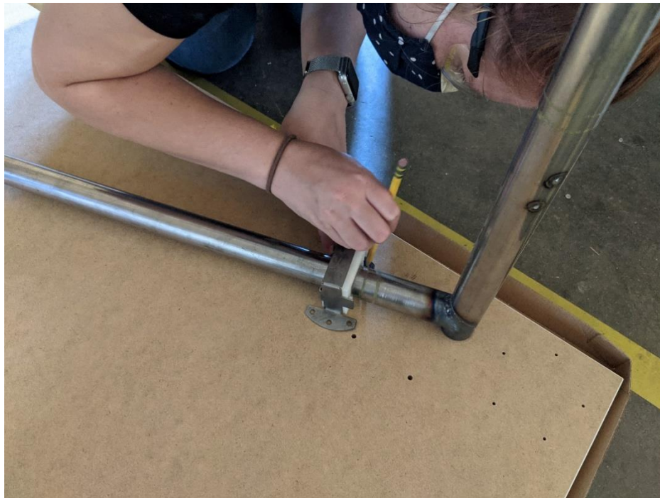
Figure Q 3: Locating the holes for wood anchors.
