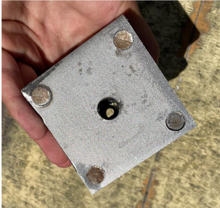
Figure 37: Checking to see if the epoxy seals between the jounce bumper and the two plates kept the inside of the jounce bumper dry.
