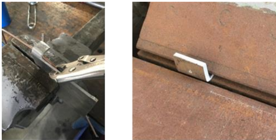
Figure 99. Bending of Follower Frame with Welding Wire
