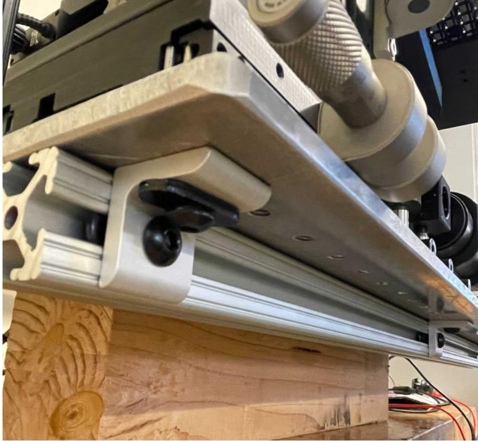
Figure 31 80-20 support beams in installed location
