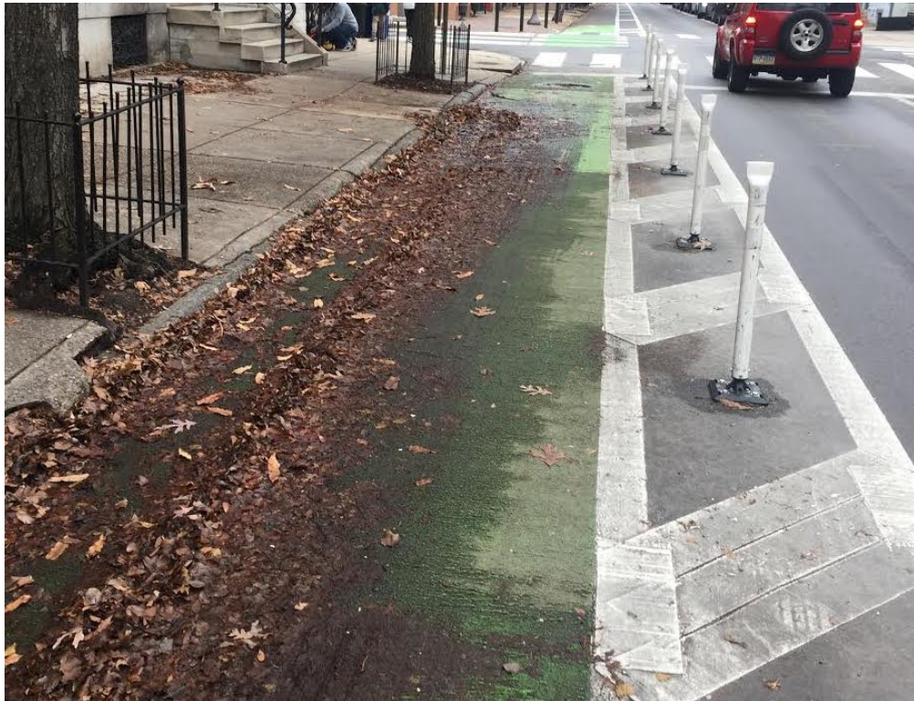
Figure 4.21: Debris Blocking the Bicycle Lane in San Francisco, California
