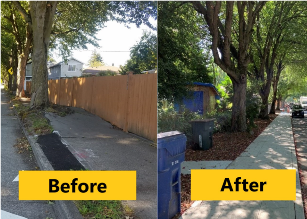
Figure 4.15: Sidewalk Improvements in Seattle, Washington
