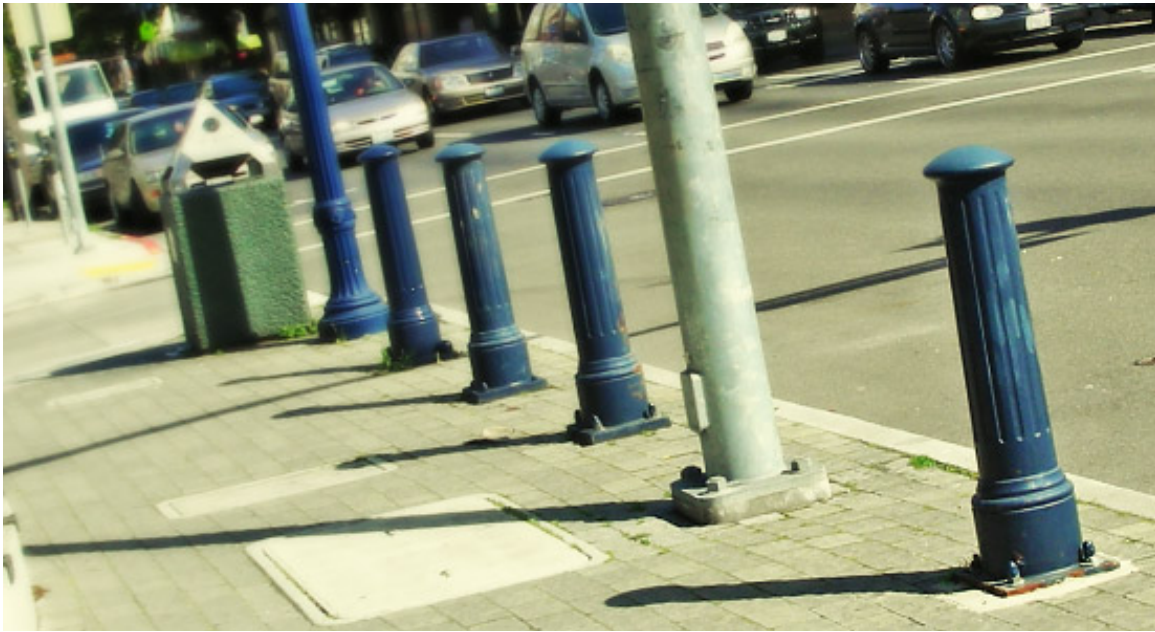
Figure 4.18: Bollards Separating Sidewalk from Street in San Francisco, California
