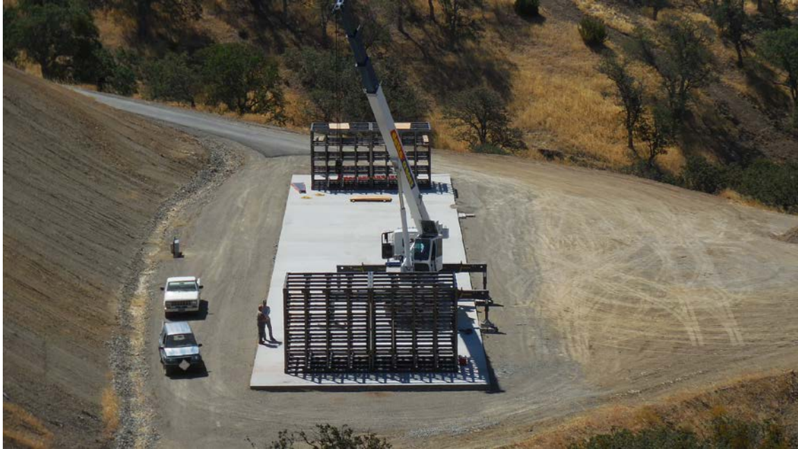
Figure 7: Modules being delivered to the test site.
