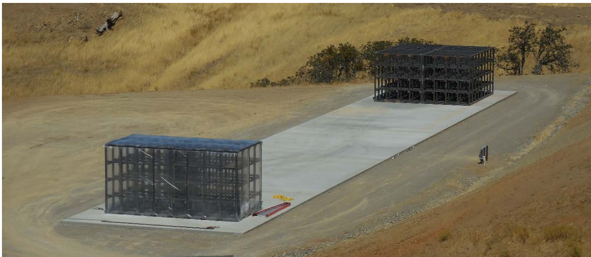
Figure 8: First modules on the test site.
