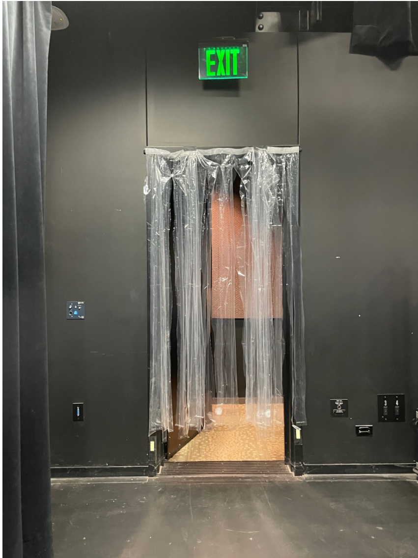
Figure A.7: The exit for A.L.I.C.E. performances. A plastic shower curtain was cut into strips and secured to the doorframe with Velcro strips.
