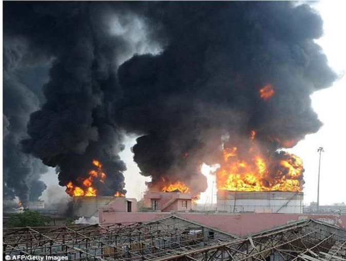
Fig. 3. Sitapura, India (2009) storage fire accident [3].
