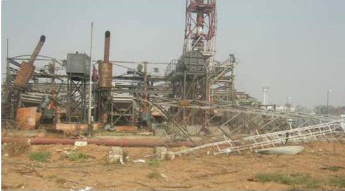
Fig. 9 Damaged Pipeline pump house from the south of the building [33]
