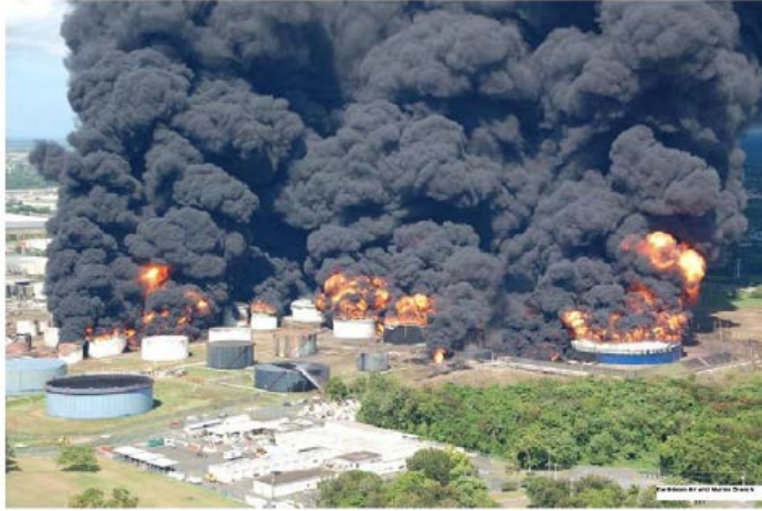
Fig. 2. Puerto Rico, USA (2009) storage fire accident [2].
