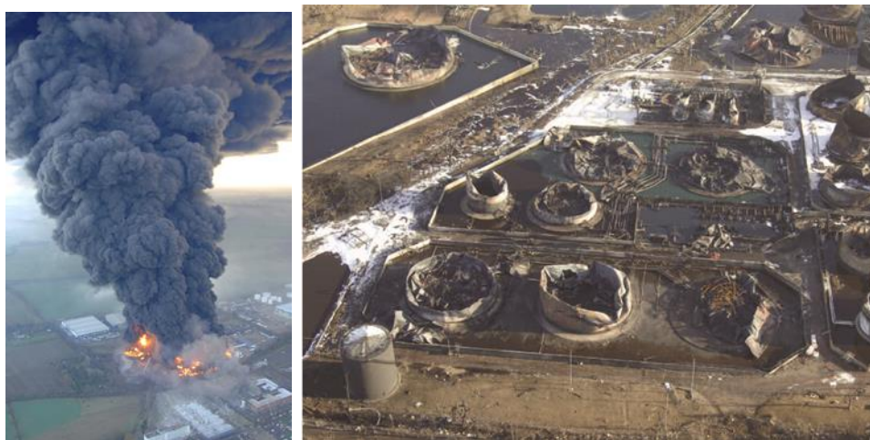
Figure 3—Images of the 2005 explosion and ensuing fire at the Buncefield tank farm.
