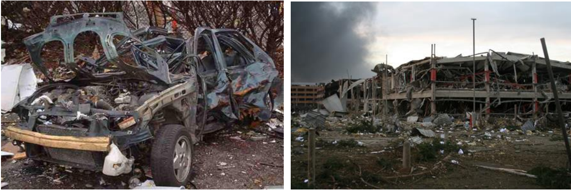
Figure 4 —Images of the damage from the 2005 Buncefield explosion: left image – automobile, right image – Fuji building.
