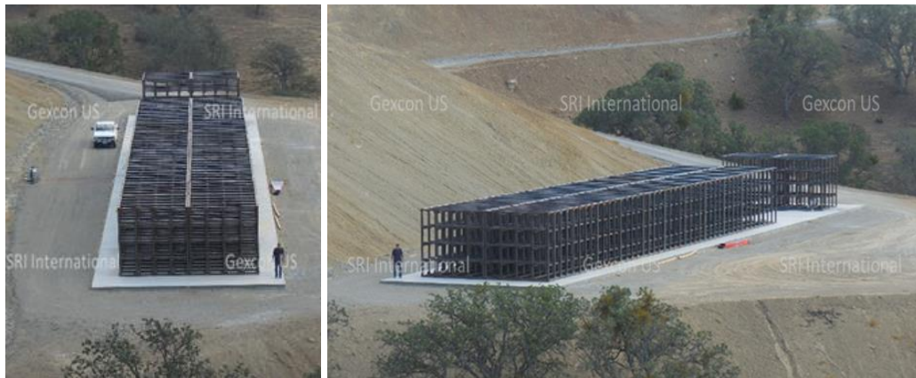
Figure 9–Finalized modules on the test site.
