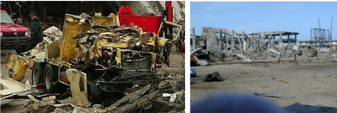
Figure 2— Images of the damage from the 2004 Skikda explosion: left image – truck, right image – maintenance building.
