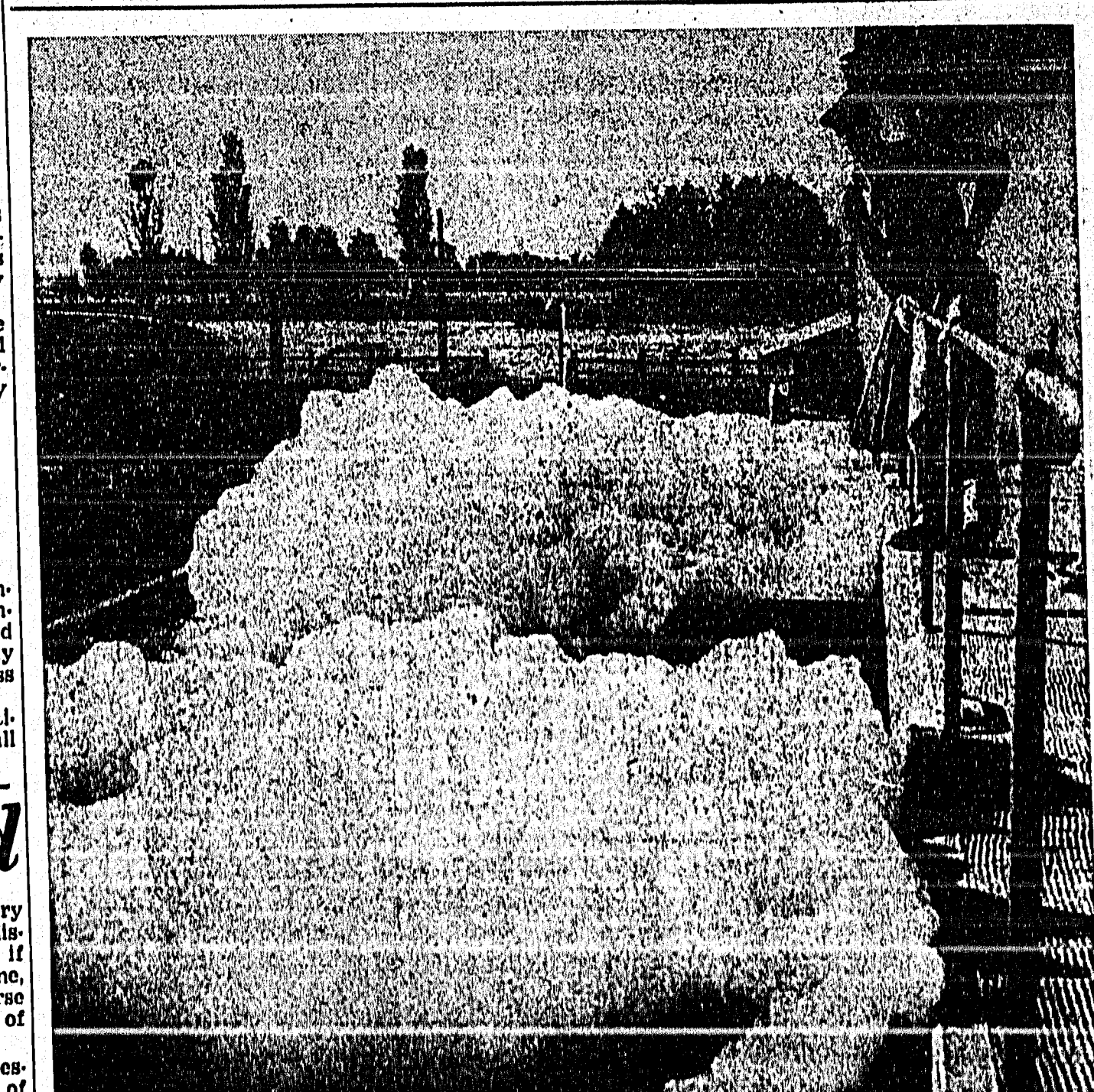
SPARKING MOUNTAINS OF DETERGENT suds which appear daily at the sewage disposal plant would seem to indicate that Pentictonites are certainly clean people. The foamy stuff is at its best about 7.30 a.m. and on washday. Monday, it will reach a height of six or seven feet. The detergents in the sewage are churned up during the disposal process and on a windy day it is not unusual to see small, white "clouds" floating around the neighborhood. Plant assistant Alex Forsyth, shown above, finds the suds a bit of a problem for they must be hosed down from the walkways and equipment.
